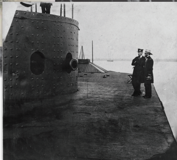
Figure 3. View on deck of the USS Monitor while in the James River, Virginia, 9 July 1862. The turret, with the muzzle of one of Monitor's two 11-inch Dahlgren smoothbore guns visible, is at left, with the armored pilothouse beyond. U.S. Naval History and Heritage Command Photograph
