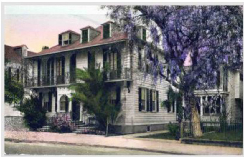
McCrady House on South Battery Street, Charleston, S.C.
